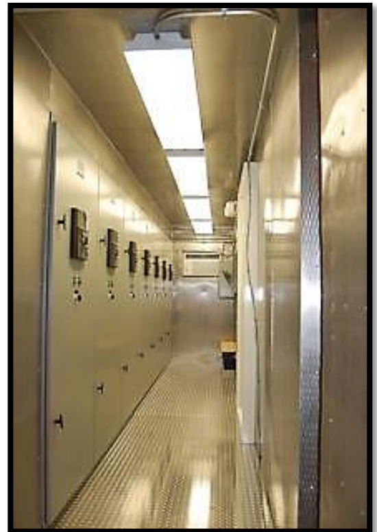
Figure 6: 20' Inside ISO Container-Based Walk-in Switchgear Module
