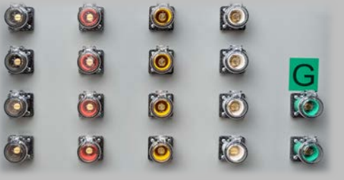
Figure 4: Male Cam-type Receptacles & Covers*
